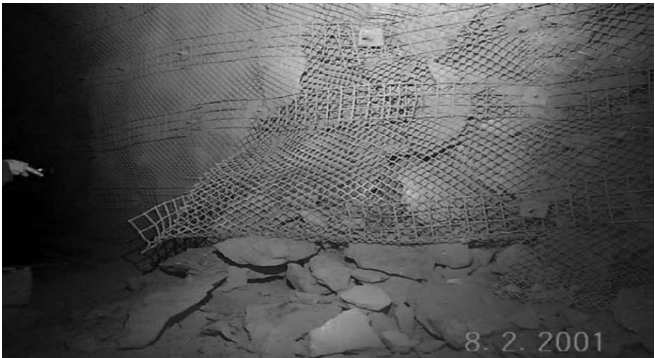
Fig: A fault-slip rock burst in a deep metal mine (Simsler, 2001).
