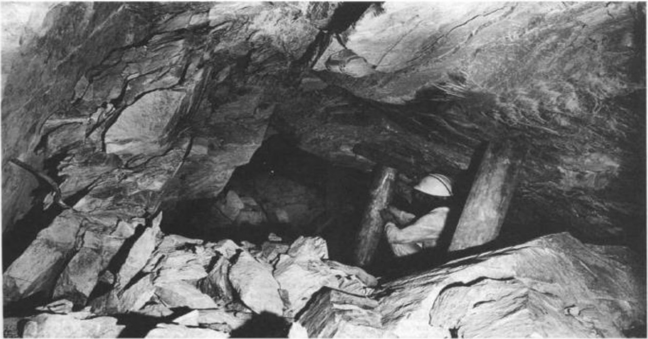
Fig: Collapse of roof arch of haulage in quartzite at depth of 2700 m after seismic effect of 2.1 M L
